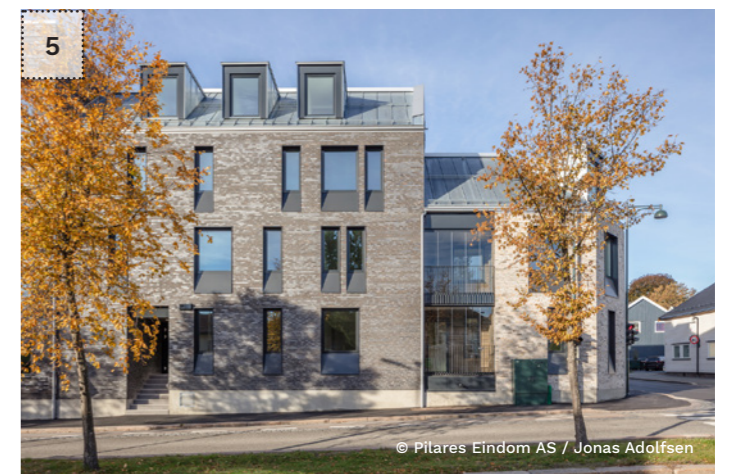
Ground floor flats could also be provided in busier locations with the building line close to the street by using a raised floor level to ensure sufficient privacy to the residents.
