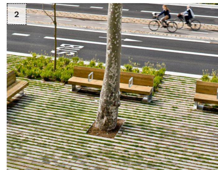
Permeable paving strategically placed within appropriate ground conditions
