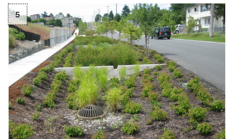
Sustainable urban drainage and rain gardens incorporated into the streetscape and public realm landscape help to deal with attenuation and limit sedimentation and pollution
